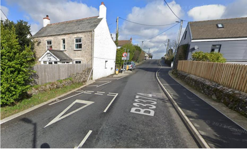
Example: Priority working in accordance with TSRGD, St Austell
