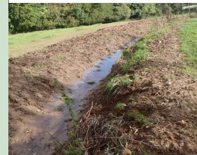
A well maintained ditch allowing a free flow of water
